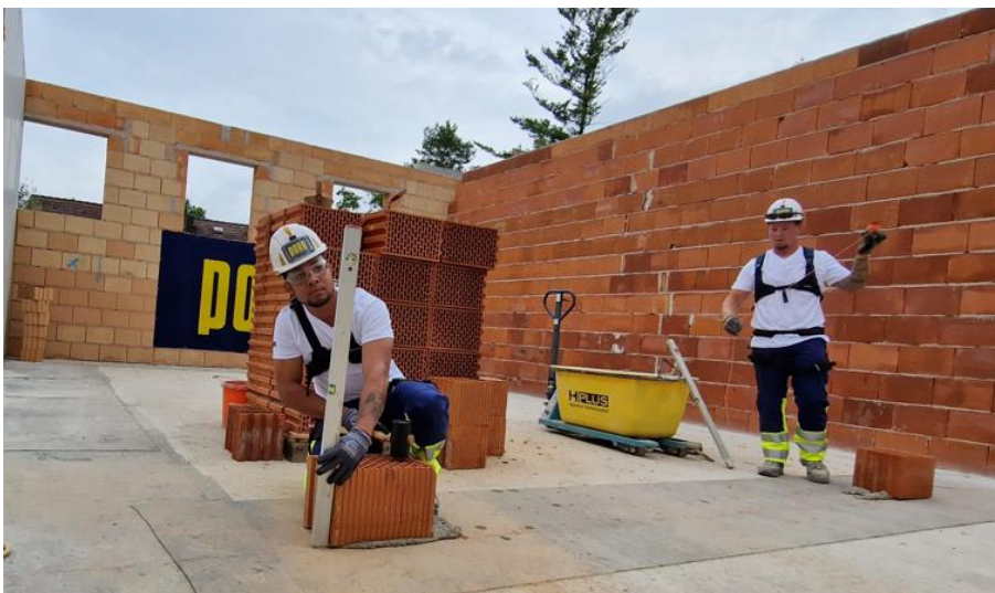
Exoskeletons help with lifting bricks on the pilot construction site © PORR
