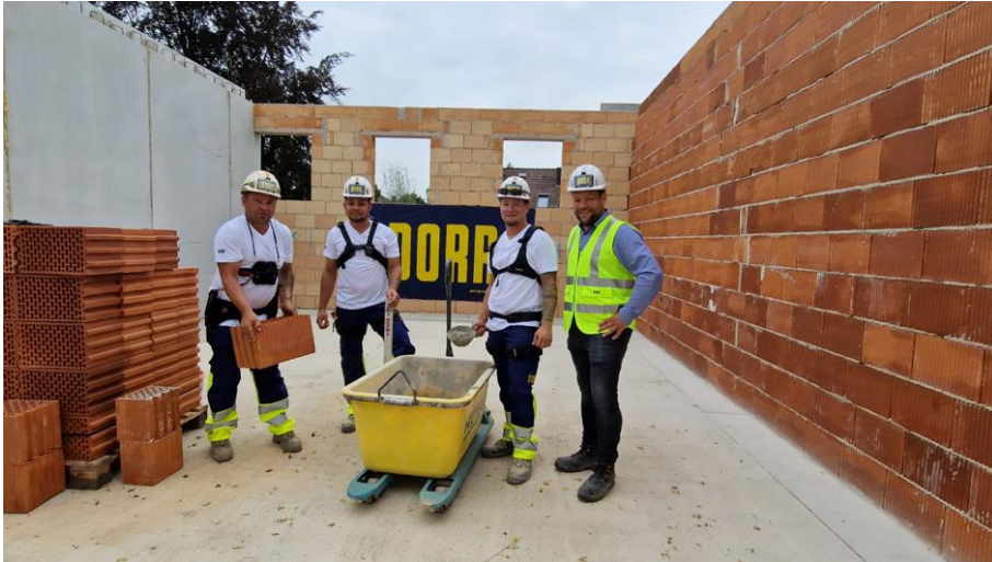
Exoskeletons help with lifting bricks on the pilot construction site © PORR
